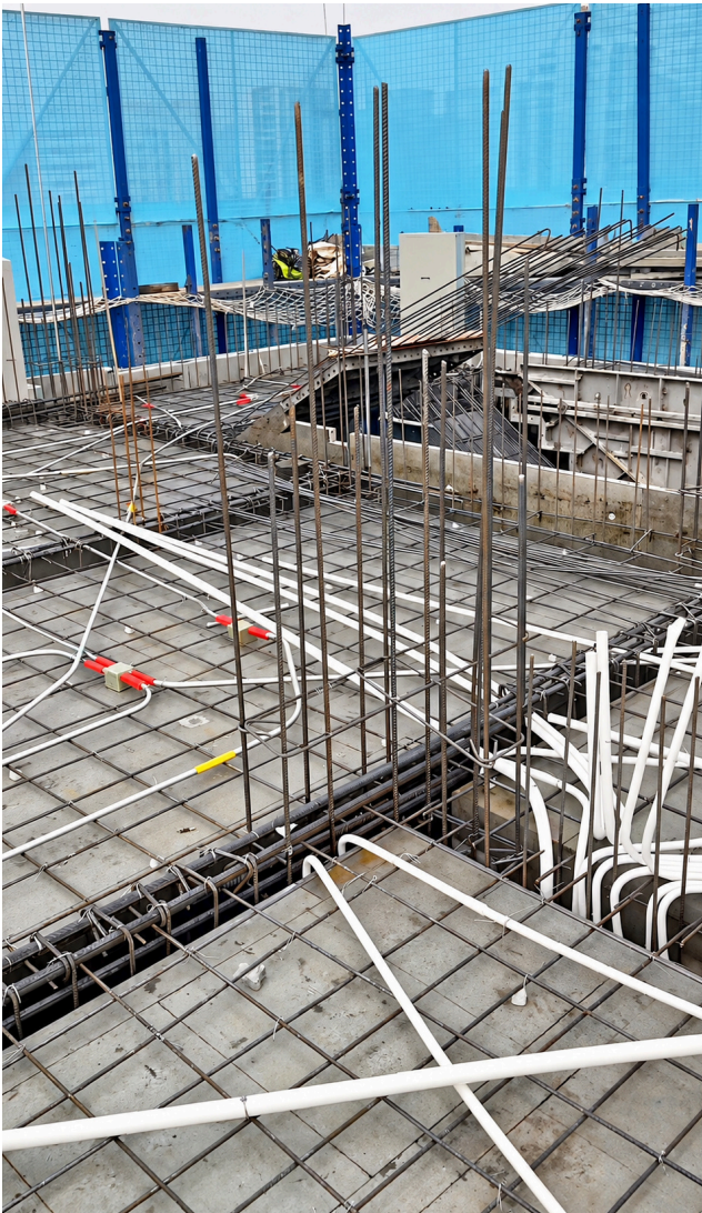
Conduit embedment during structural construction
