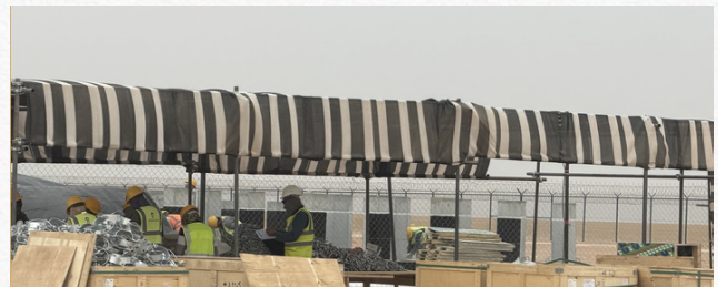
Cable drum storage and material preparation
