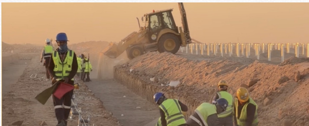
Cable pulling and roller setup
