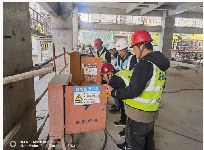
Site equipment inspection
