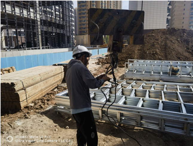
External site inspection
