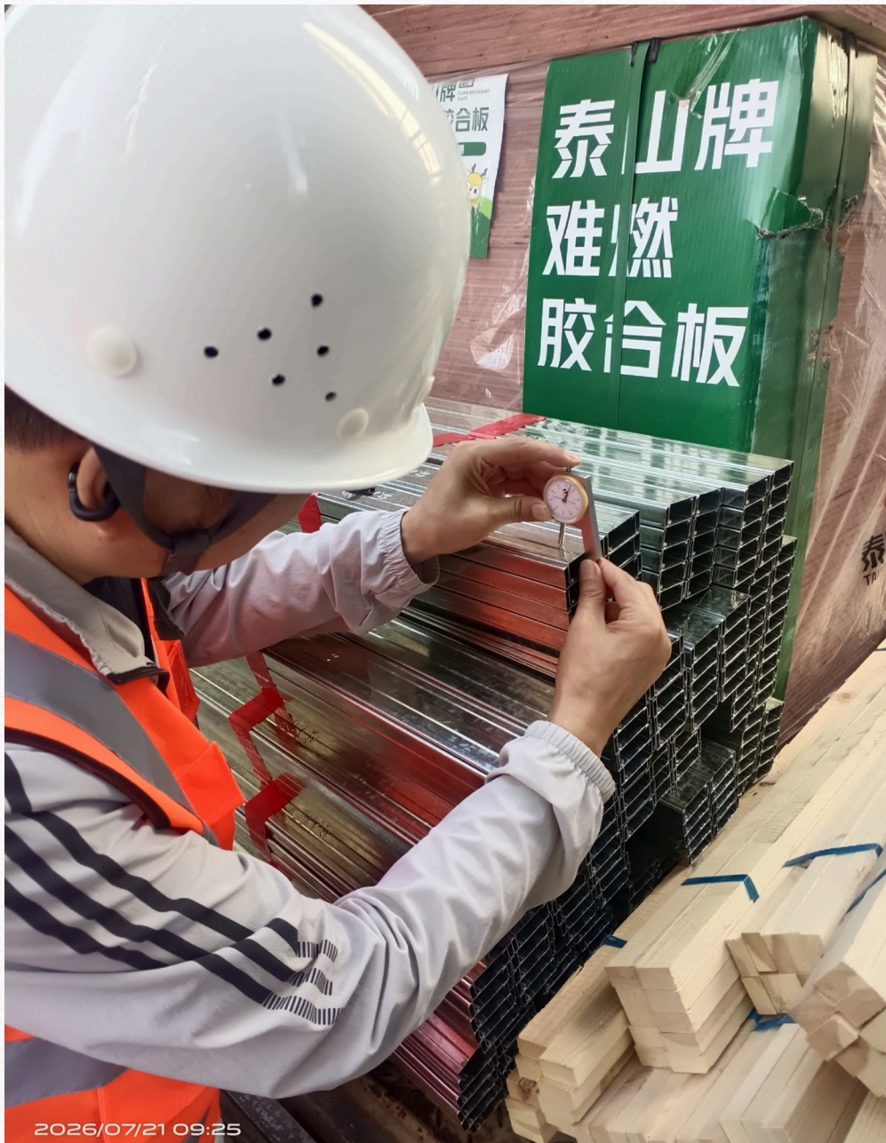
Panel dimension checks and site quality inspection
