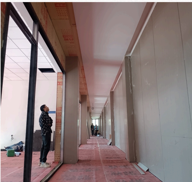
Corridor finishing works
