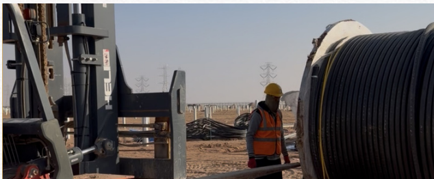
Forklift handling of cable drums
