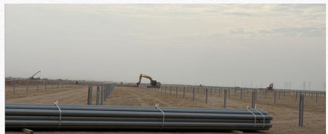
Pile and structural material preparation
