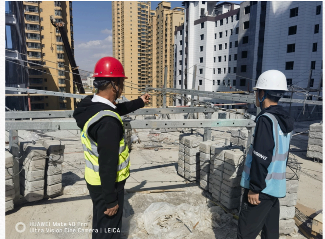
Site construction coordination
