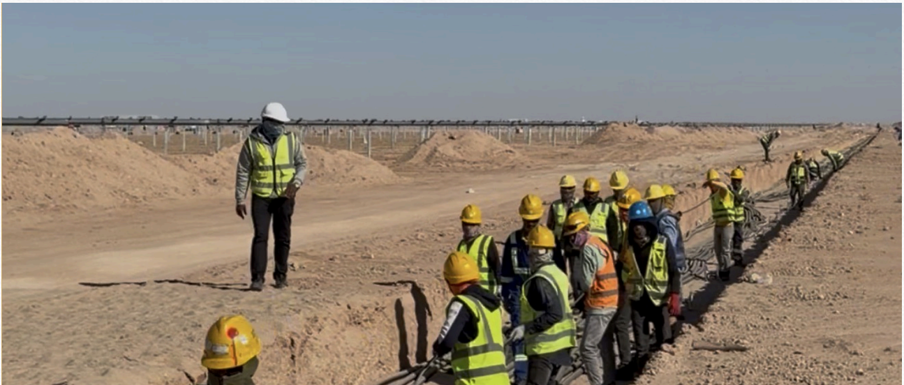
Cable installation and crew coordination
