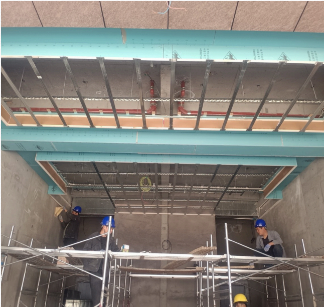
Ceiling installation
