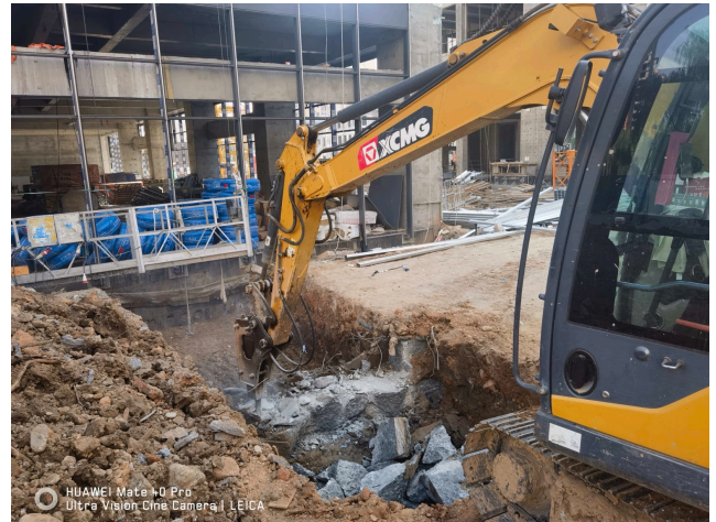
Earthworks and mechanical breaking
