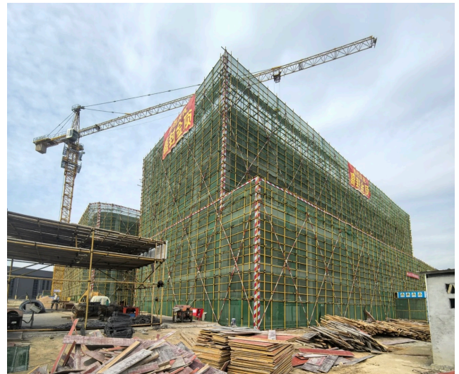
Structural works and scaffolding
