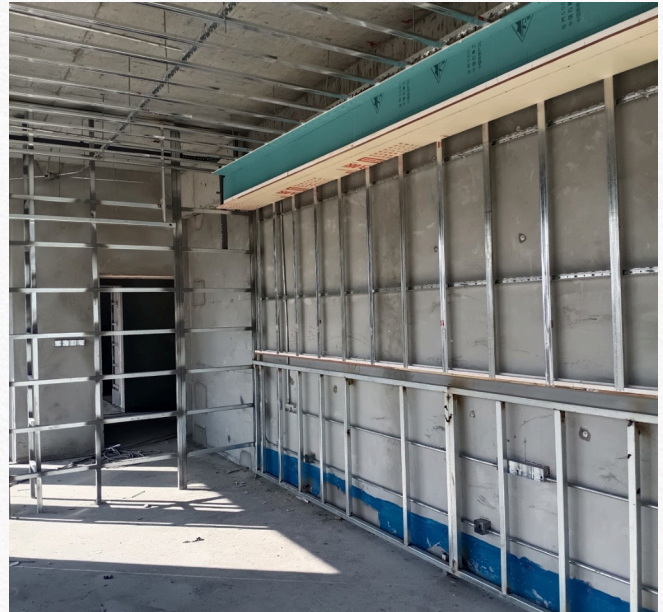
Partition framing installation
