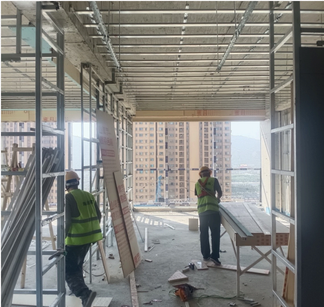
Interior construction site
