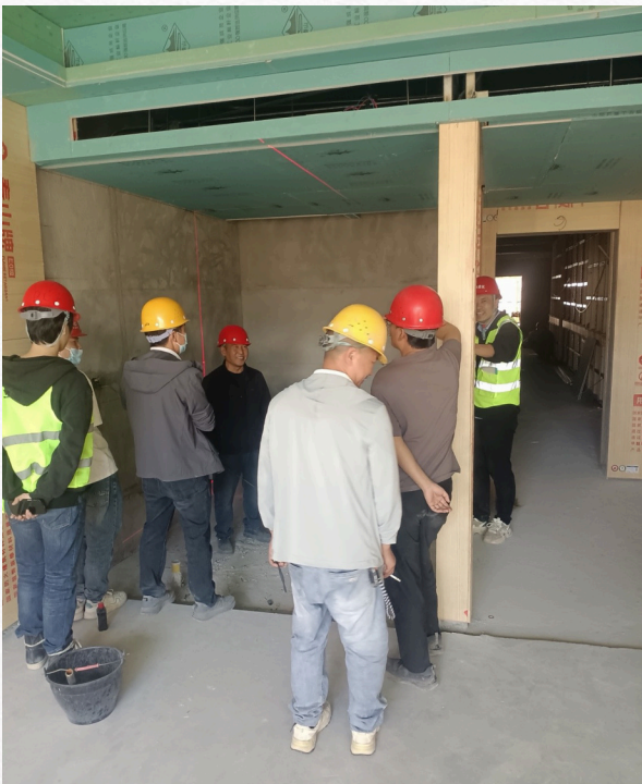
Interior construction inspection
