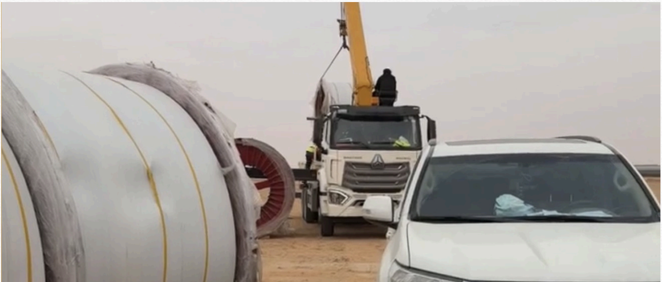
Cable drums and lifting resource coordination
