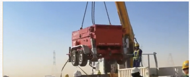
Equipment lifting and relocation
