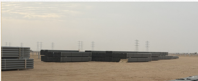
PV structural material storage
