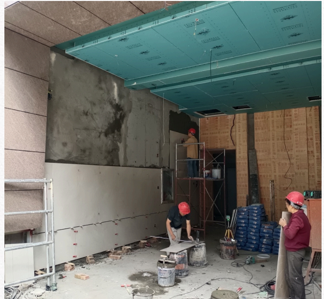
Interior fit-out works
