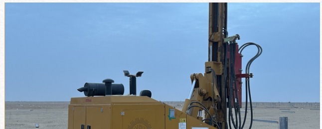
Solar piling equipment
