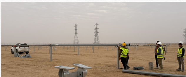
Beam installation and inspection
