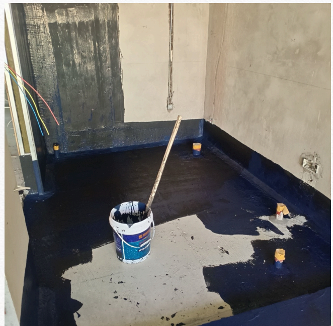
Interior waterproofing
