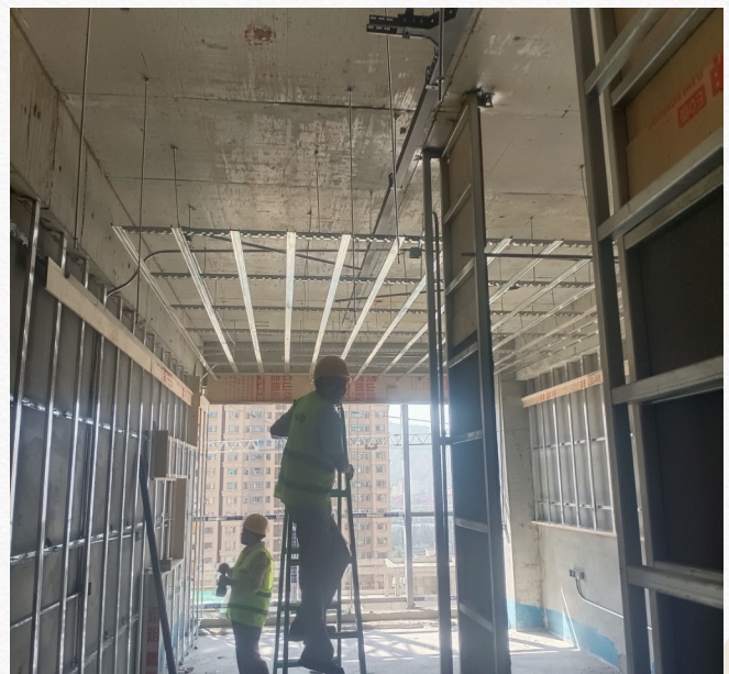
Ceiling framework construction
