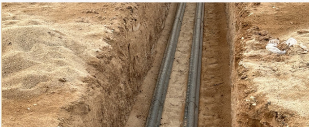
Cable laying inside trenches
