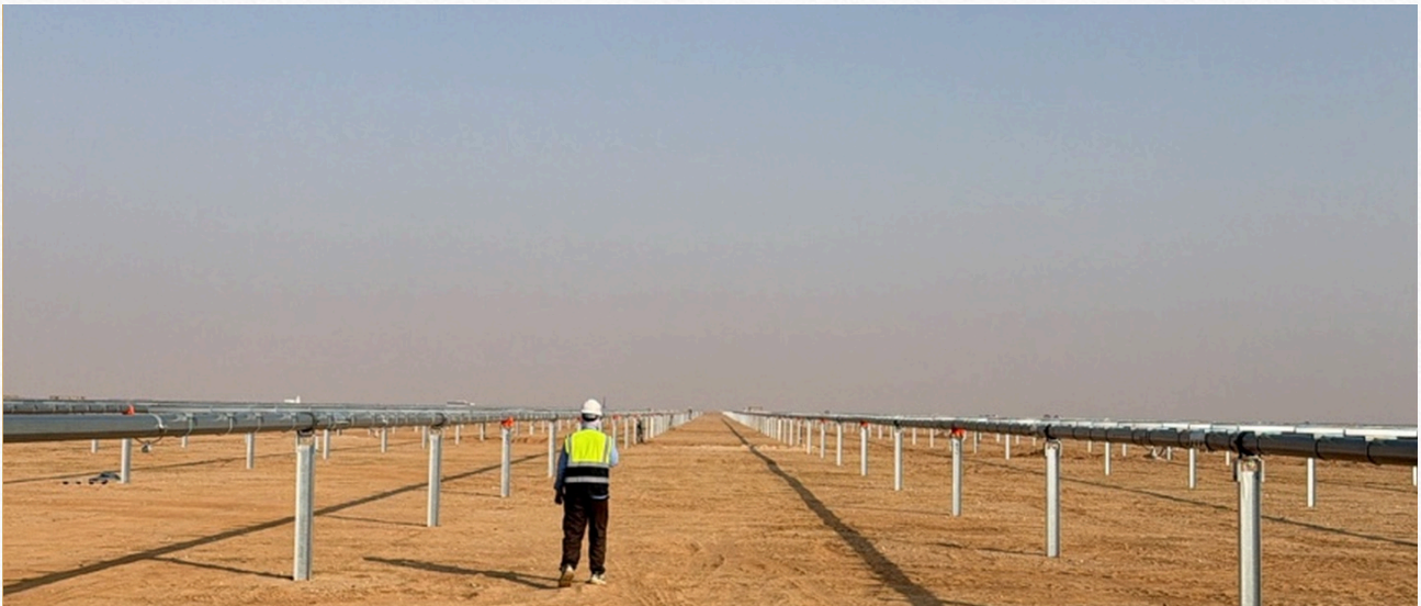
PV mounting structure construction
