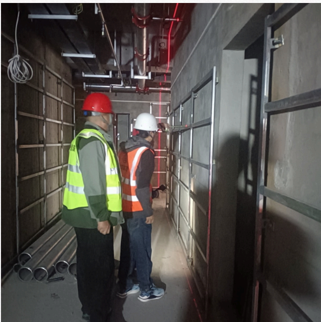
Pipework site inspection
