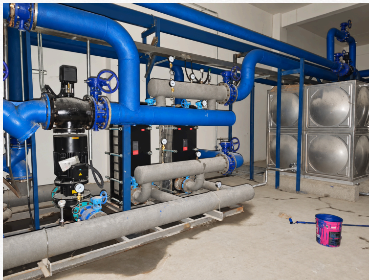
Plant room pipework and equipment installation
