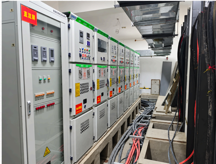
Distribution equipment and cable installation
