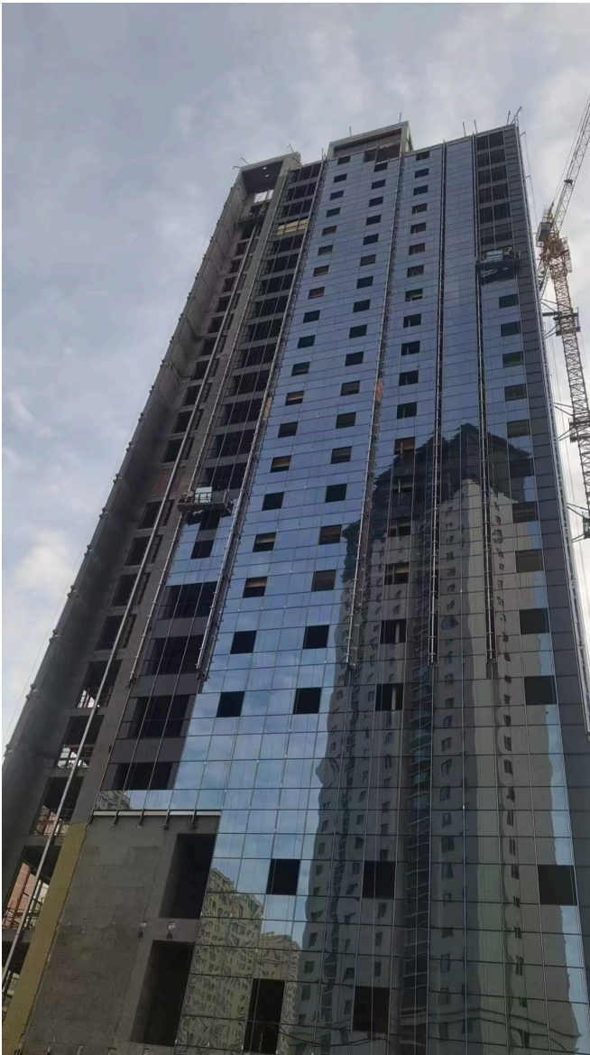
Building exterior and facade works
